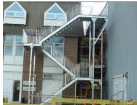
Galvanised Fire escape built to BSEN 1090 specification
